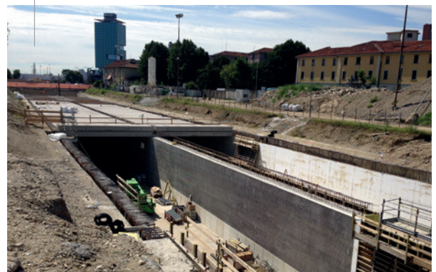
ZARA-EXPO Tunnel, Milan Tunnel ZARA-EXPO, Milano
